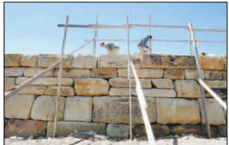
James Reid, left, and Pablo Ortiz worked atop the dry-laid stone retaining wall along Tates Creek Road this week.
